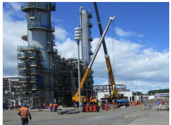
Distillation Plant – Cranes positioned for lifting equipment in/out
