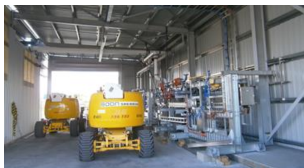
New Load-out Bay Structure
